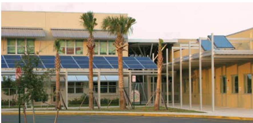
Pine Jog Elementary, School District of Palm Beach County; LEED NC Gold Certified; Zyscovich, Architects; photo courtesy of Thom Grafton.
